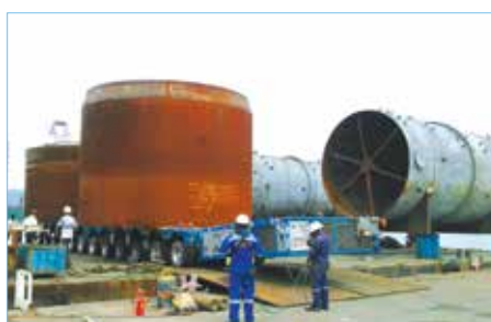
Last package being rolled onto the barge
