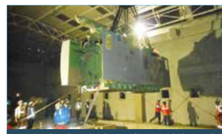
HYT's wheel Lathe being lowered through the roof onto the installation pit
