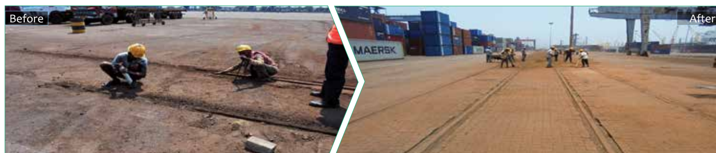
ALIGNING AND CLEANING UP RAIL TRACKS
